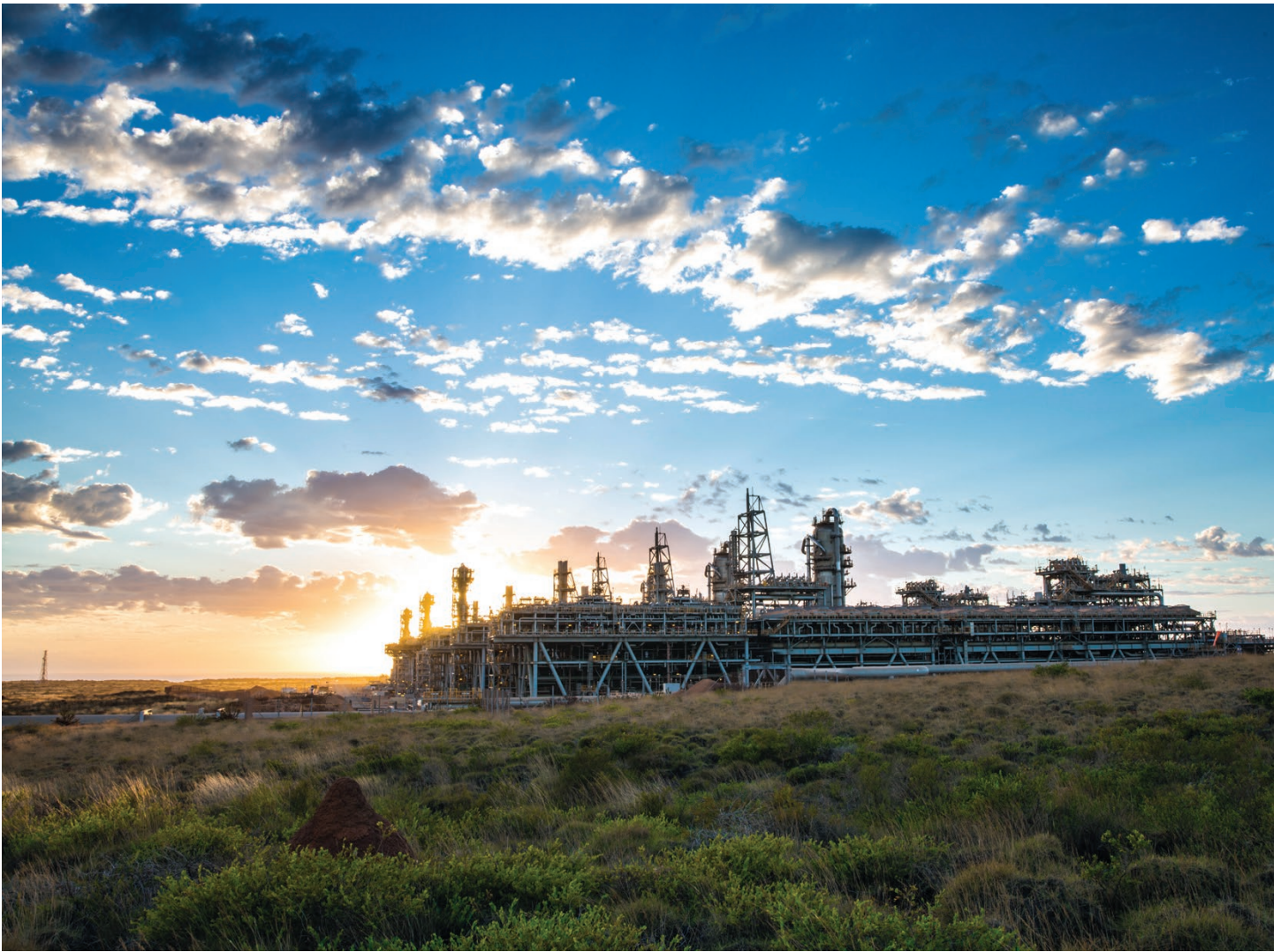
Startup of the third LNG train at the Gorgon Project was achieved in March 2017.
