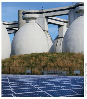
When renewable resources such as solar are coupled with batteries or other energy storage devices, critical facilities like wastewater treatment plants are able to maintain power even if the centralized grid goes down, without needing to depend on unreliable and expensive diesel generators.
